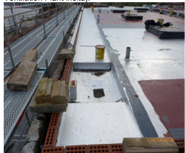
Looking South along the East Gutter (Argyle St.): Work in Progress – Laying of Roof/gutter membrane and Insulation including rebuilding of parapet wall.
