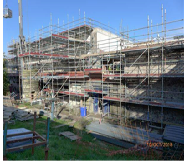
West Elevation – Rear Elevation of Building.
