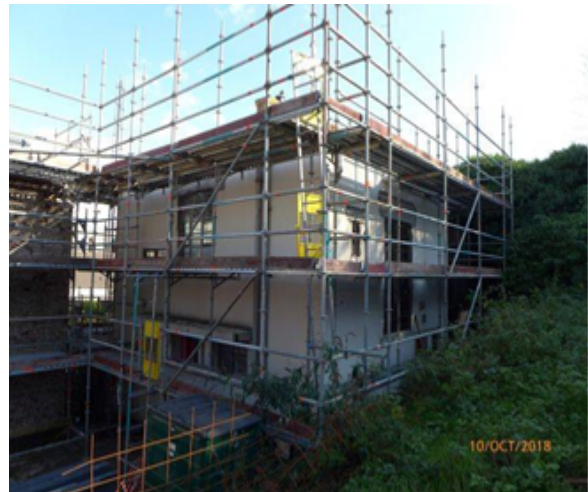
North & West Elevations – Caretakers House (NB: new windows in situ).
