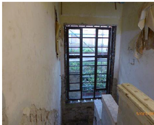
West elevation: new window to stair now installed.
