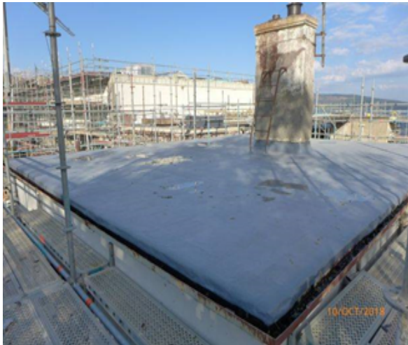
Looking North: Caretakers House Roof (NB: Fly Tower south elevation visible in background).
