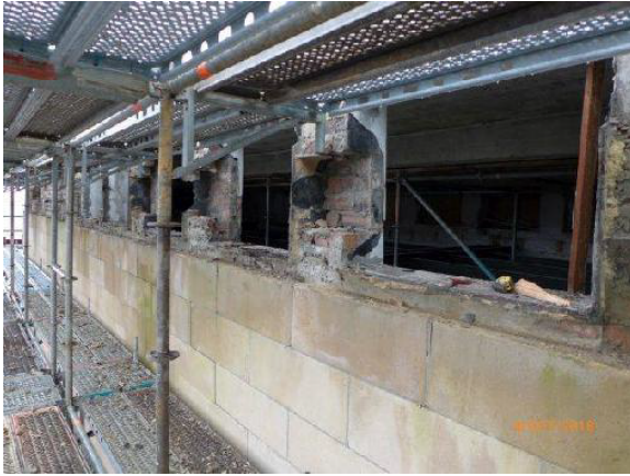
North Elevation (Mackinlay St.): Temporary window boarding removed for examination of cast stonework and backing wall.
