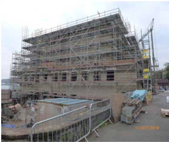
North Elevation (Mackinlay St.).
