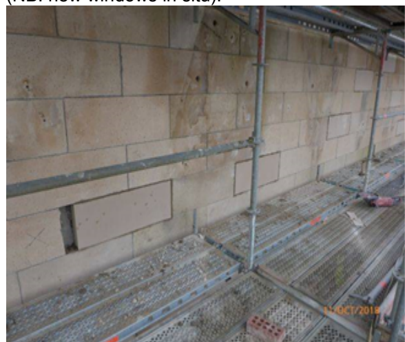
East Elevation (Argyle St.) – NB: Work in Progress: defective cast stonework replacement with new stone).
