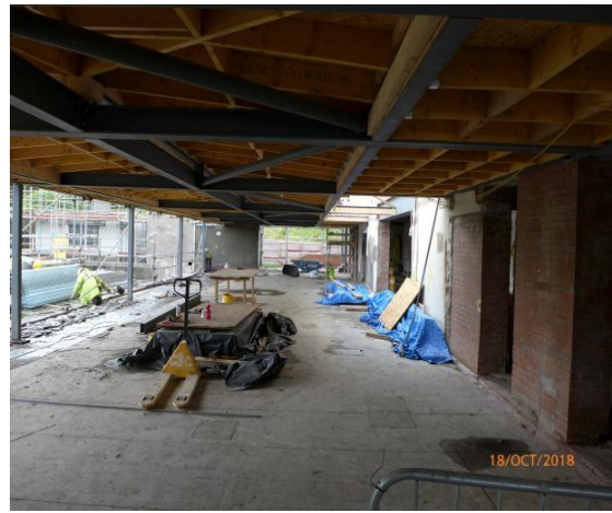
New Offices: General view looking West
