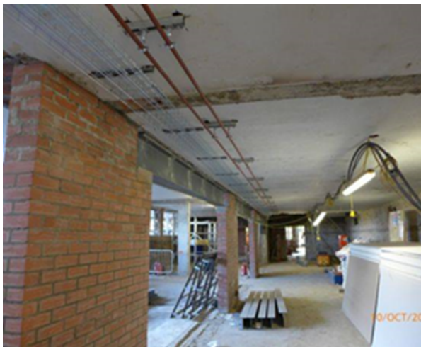
Exhibition Space: General View (NB: Work in Progress: new openings formed to increase foot print & installation of service pipework).
