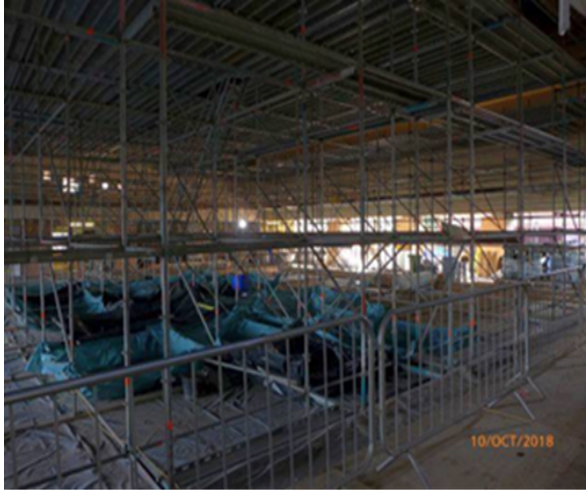
Auditorium/Main Hall: General View of Scaffold and rainwater protection.
