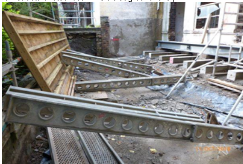
Shop Area: Work in Progress to create new extension to increase Shop floor area.
