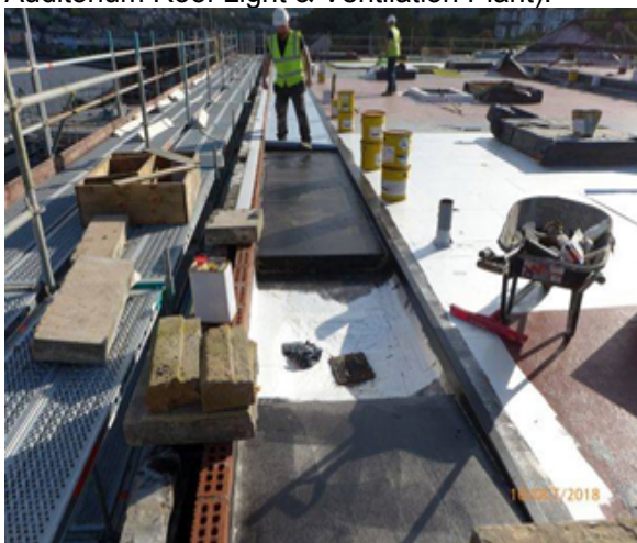
Looking South along the East Gutter (Argyle St.): Work in Progress – Laying of Roof/gutter membrane and Insulation including rebuilding of parapet wall.
